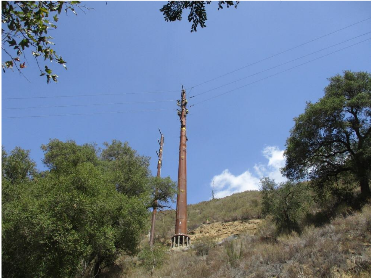
Photo 3: Crews were observed sagging and dead-ending wire at Z118096 (TL 682).
