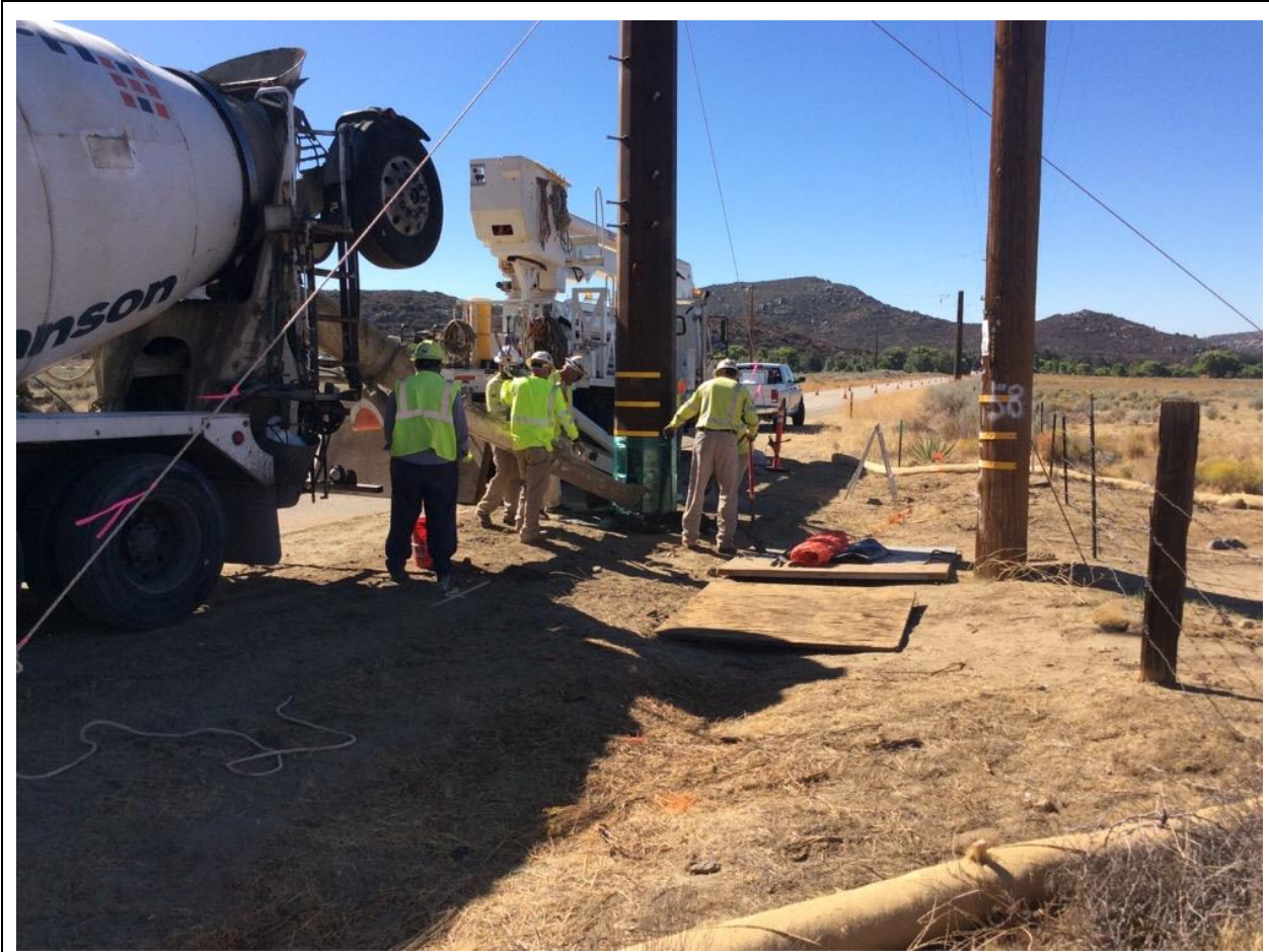
Photo 1: Crews were observed setting pole bases along TL 629C.
