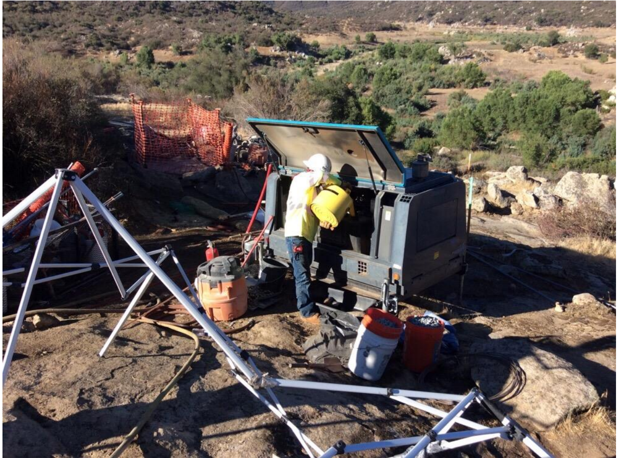
Photo 6: In accordance with the CFPPP, the generator at P258090 was fueled first thing in the morning after it had cooled overnight. In addition, a drip pan was staged under the fuel can to prevent potential spills or drips onto the ground during fueling in accordance with MM PHS-2.
