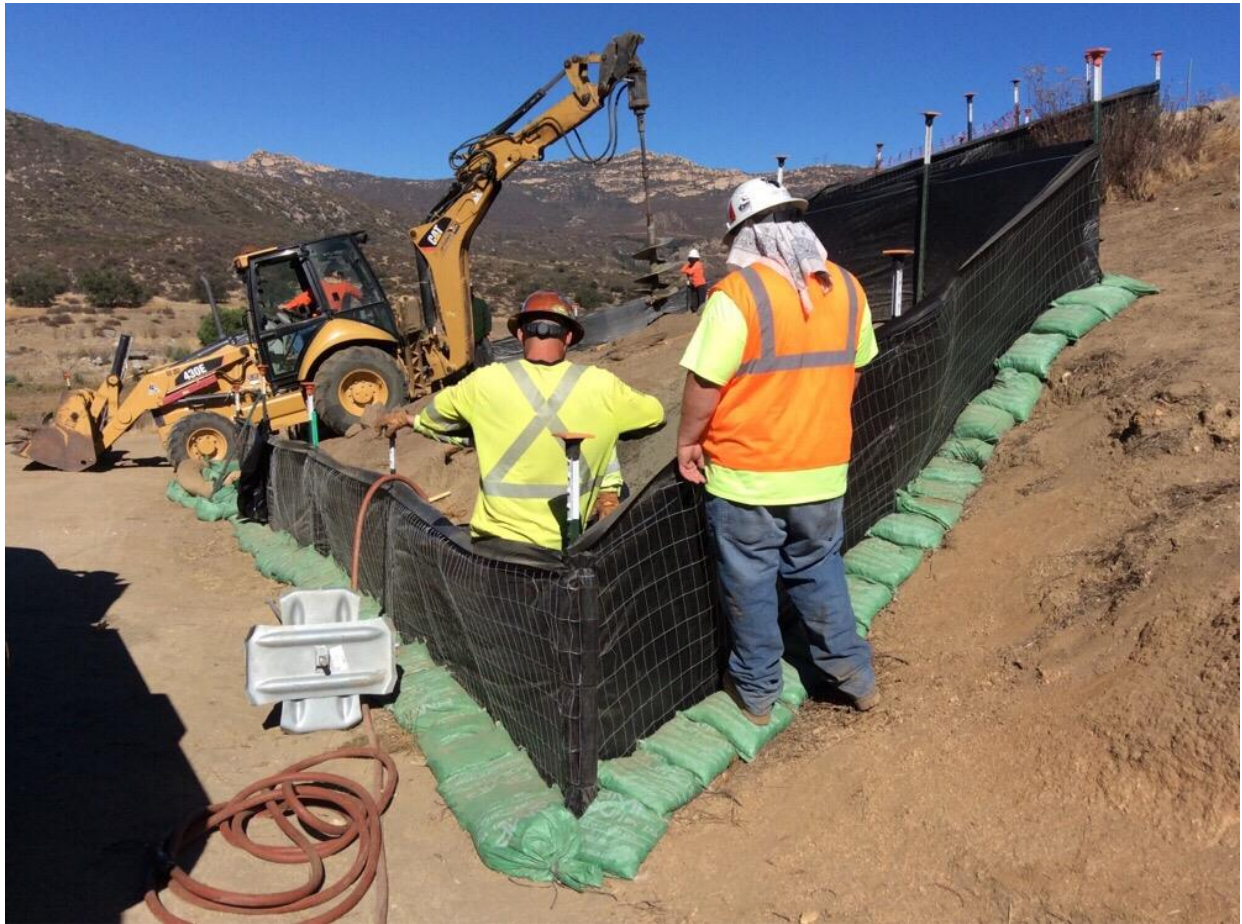
Photo 5: Arroyo toad exclusion fencing was installed at P258086 (C157) in accordance with the Arroyo Toad Monitoring and Relocation Plan (MM BIO-33).
